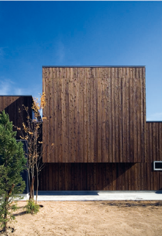
architect/Takanobu Kishimoto (CONTAINER DESIGN) photo/Eiji Tomita
